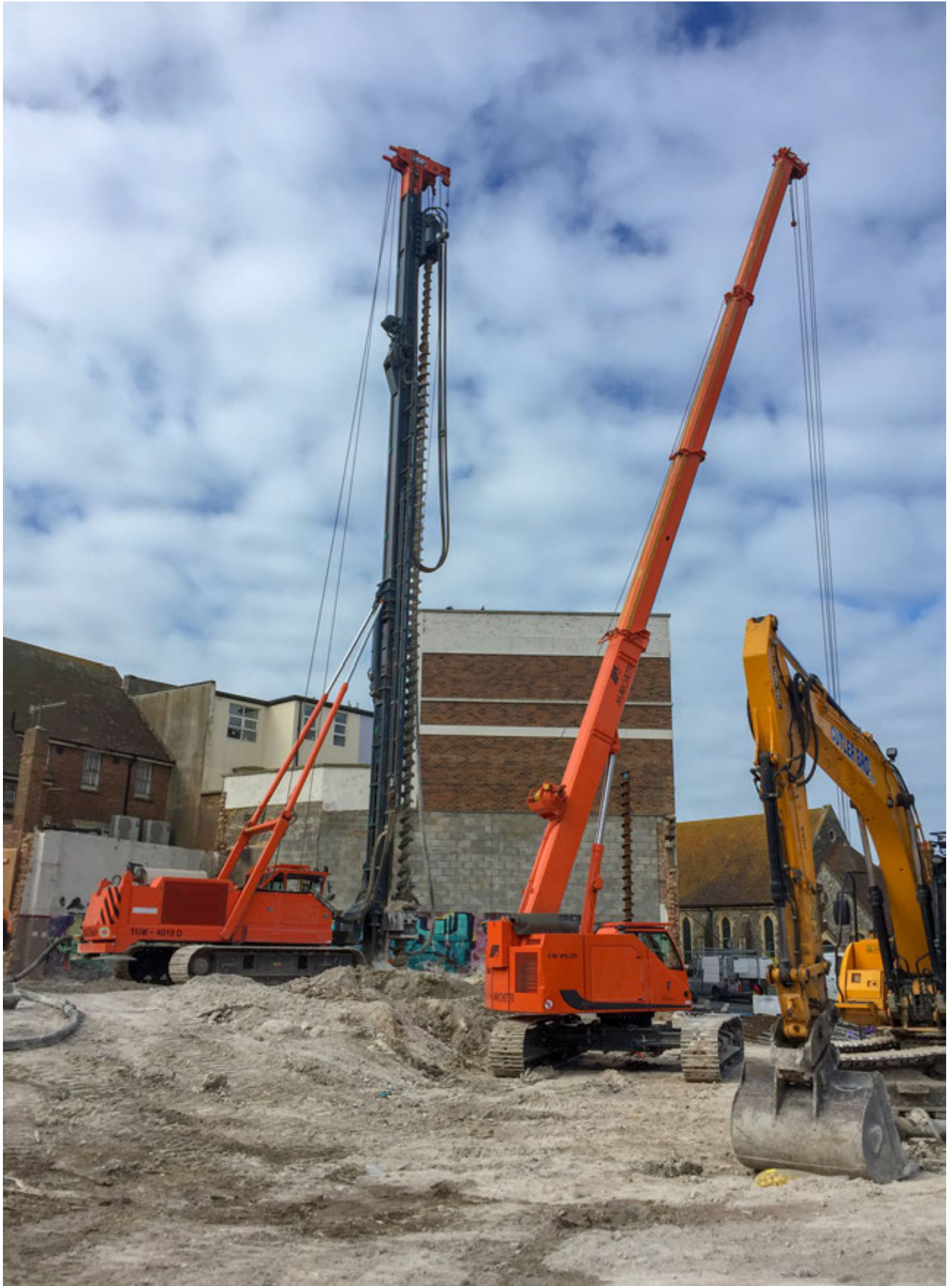
CFA piling in progress
