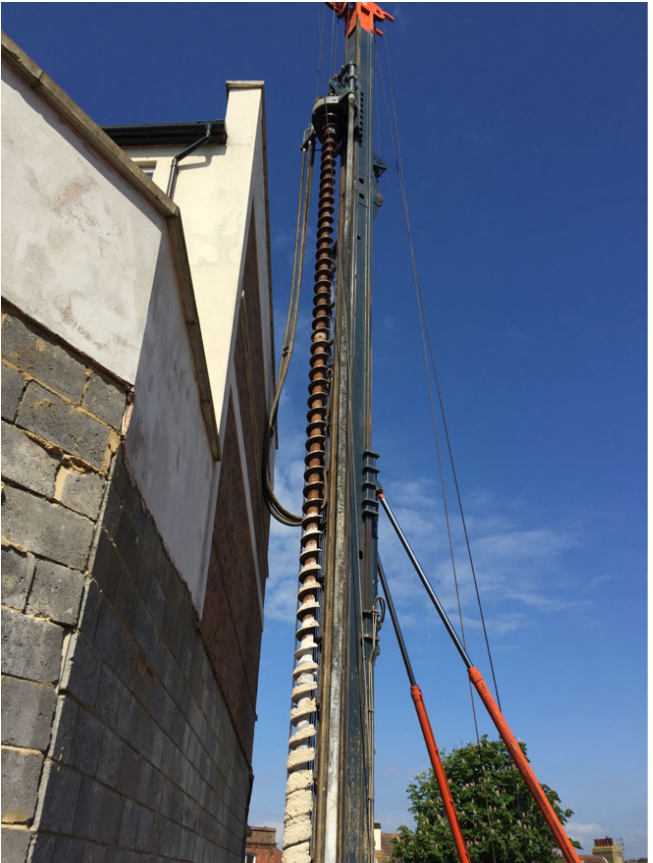
Working in proximity to adjacent structure
